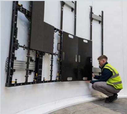
Pre-assembled mounting components to reduce on-site installation time
